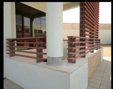
The composite timber fins can be fitted horizontally or vertically
